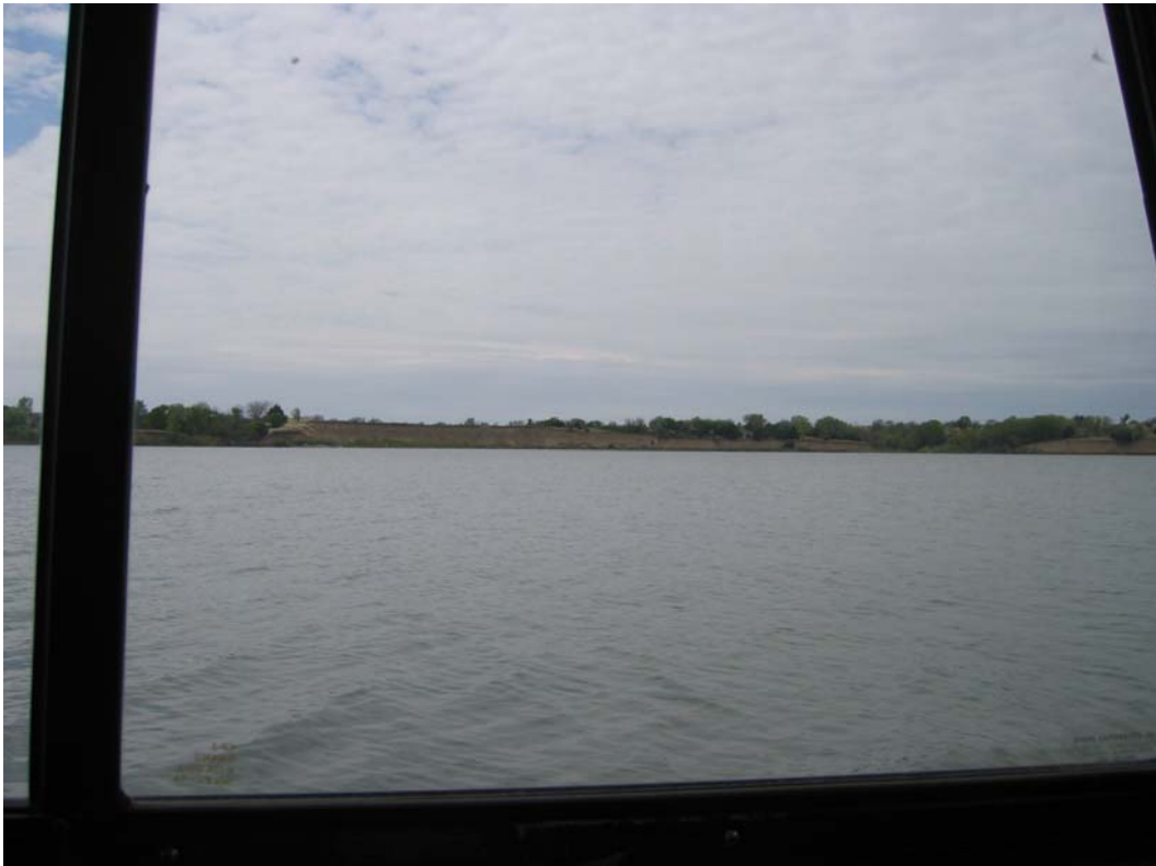
Figure 6 - View of shoreline erosion over extensive area of reservoir.
